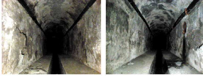
Fig. 13.13: Alert ID 1. This alert was generated as evident defects on the left wall can be found (right with the rear camera). Also sediments on the floor had been detected. Images obtained from front camera (left) and rear camera (right). Location: 41.386359^{\circ}\text{N} , 2.183163^{\circ}\text{E} . Local Time: 2017-10-17 10:58:15
