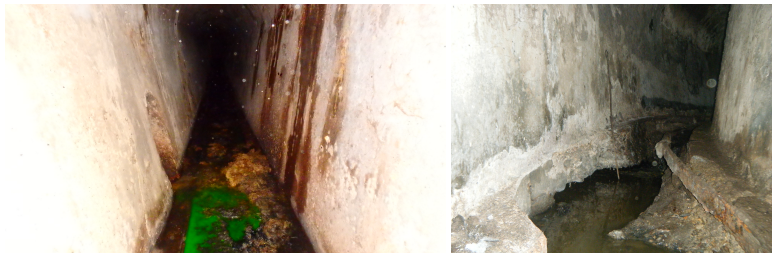
Fig. 12.11: Examples of sewer defects. Left: serviceability of sewer compromised by sediments. Right: structural viability of the sewer affected by sinkhole on the ground.
