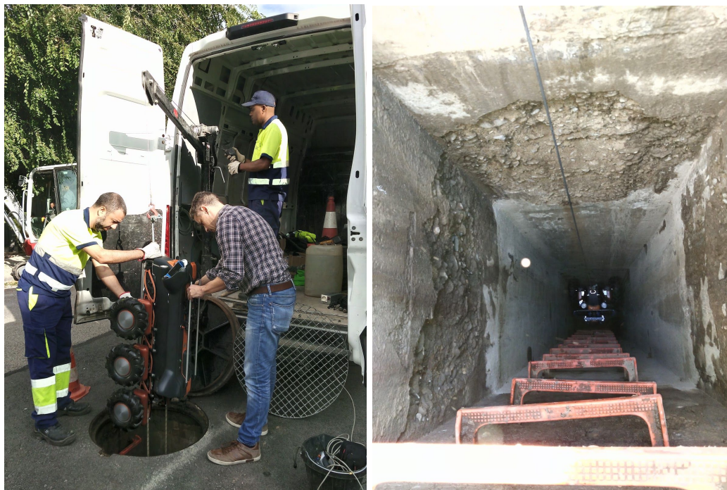
Figure 3.1: Top: the new SIAR platform on one of BCASA's vans. Bottom: the robot is deployed into sewer through a 10-meter manhole.
