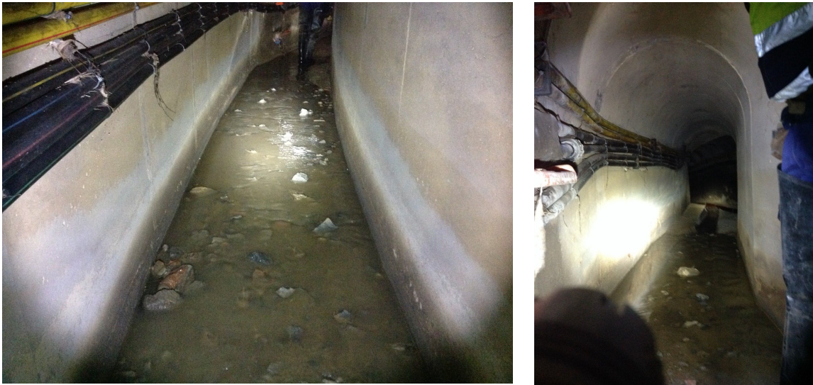
Figure 2.4: (Left) Sediments in the middle of segment 3. (Right) The sediments end just before reaching segments 4 and 5.
