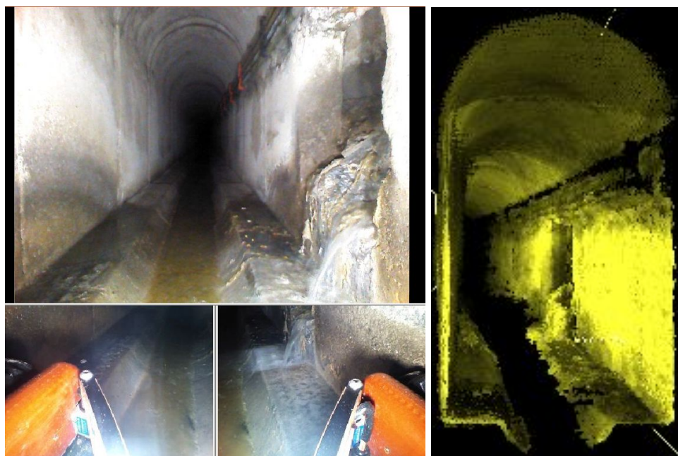
Figure 5.9. Left: Composed snapshot of three frontal cameras in the Structural Element 1. Some sediments under an inlet over the rightmost curb can be found. Right: 3D mesh obtained from the sensors, where metric measurements can be done (the estimated height of the inlet over the curb is of 0,191 m).
