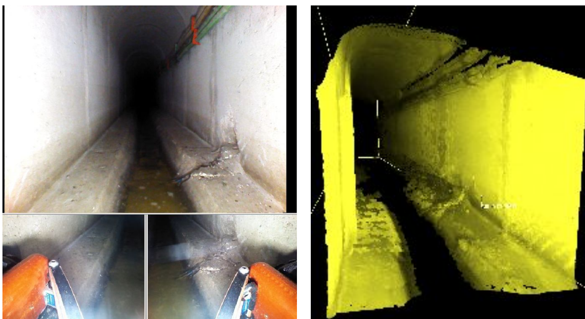
Figure 5.10. Left: Composed snapshot of three frontal cameras in Structural Defect 2. The defect is found in the rightmost curb and is composed by sediments that come from an inlet. Right: 3D mesh obtained from the sensors. The height of the sediments is estimated in 0,072 m.
