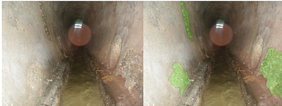
Figure 15: Left: sample of a textural defect that will be used to train a deep neural network for detection of its own kind. Right: manual labelling of the regions where the defect is present in the sewer's walls.
