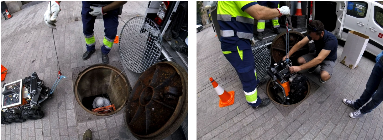
Figure 11: Frames of the video in which the deployment operation is shown.
