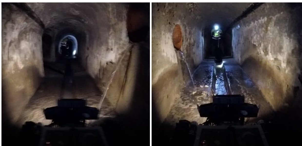
Figure 2.30. Small dirt water falls from the walls.
