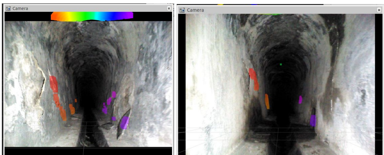
Figure 6.14: Overlaid on the original images some candidate zones of defects are shown. Left: some cracks on the floor and left wall can be seen. Right: a deformation on the left wall is highlighted, as well as a hole on the right (in this case, an inlet).
