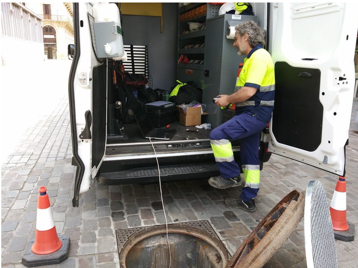
Figure 2.9. An operator from BCASA safely guides the robot in assisted teleoperation mode from the outside of the sewers.
