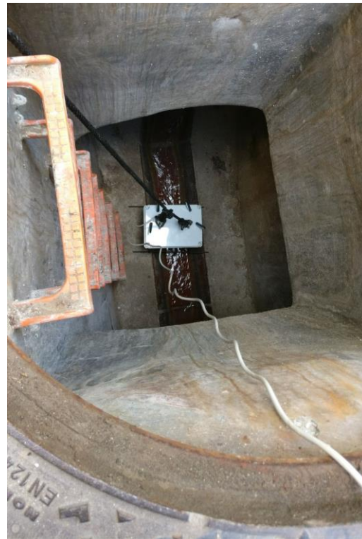
Figure 9: ARSI Wi-Fi router in its watertight case deployed in a sewer manhole
