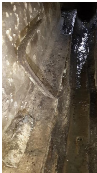
Protruding metallic rails
