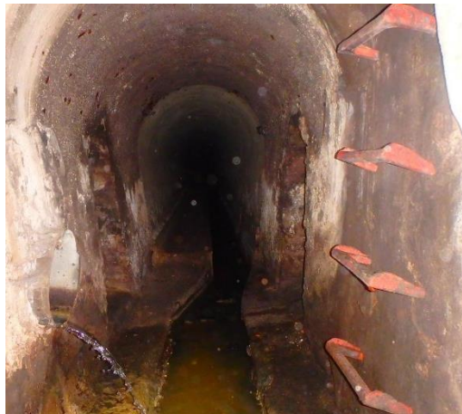
Obstacles on the sewer banks
