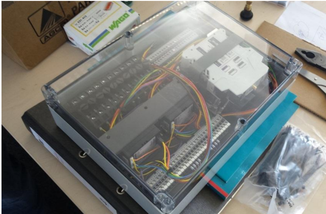
Figure 16: Electronic box with fuses, Wifi-to-CAN Gateway and Motor Controllers.
